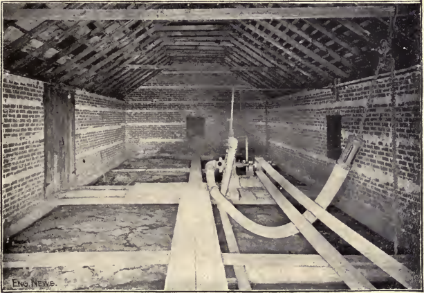
FIG. 38—INTERIOR OF CHAMPAIGN, ILL., SEPTIC TANK. (From Engineering News .)
